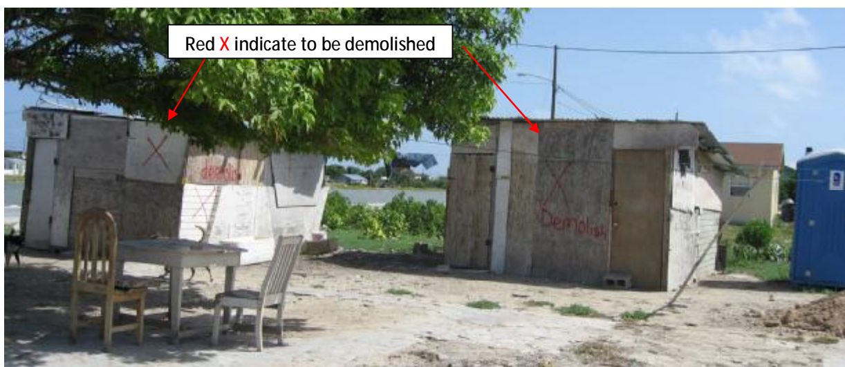
Picture 1: Houses that have been earmarked for demolition
