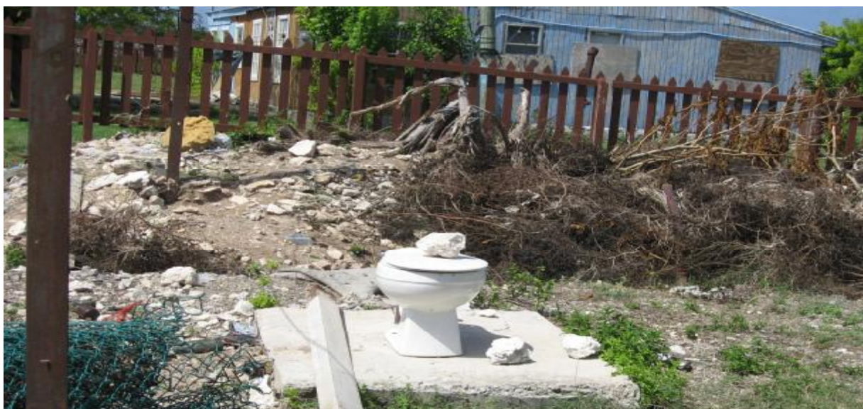
Picture 3: Bathroom destroyed during Hurricane Ike
